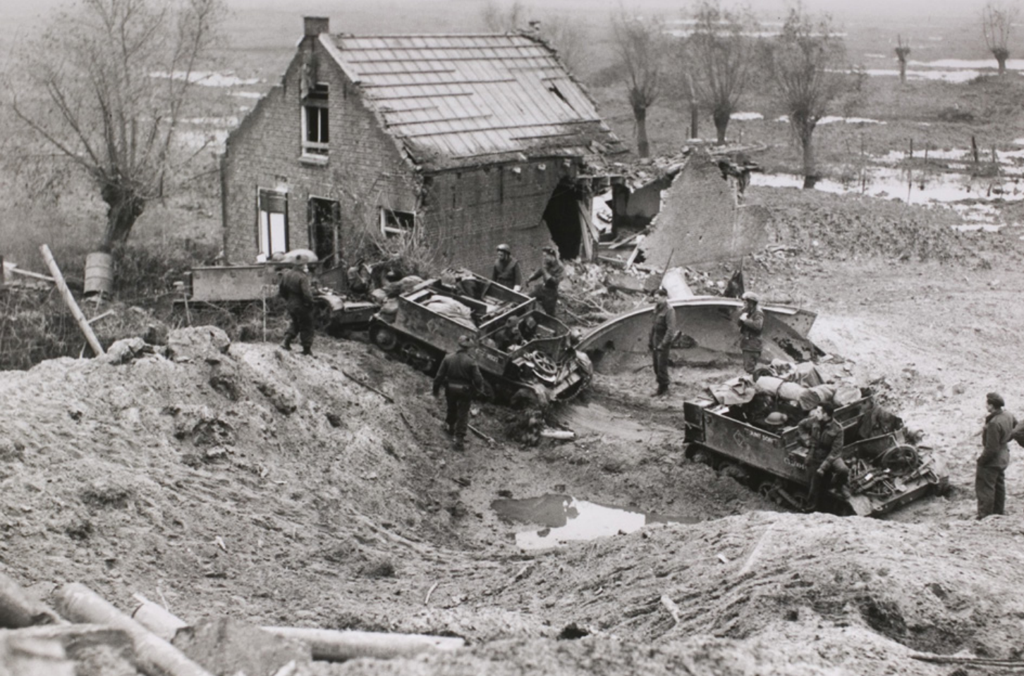
Canadian breccarriers plough through the mud near Breskens during the Battle of the Westerschelde
